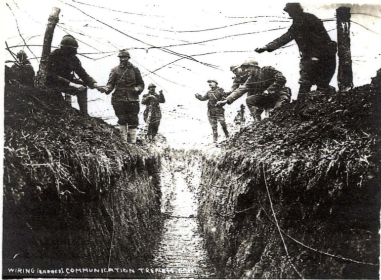
WIRING (BARBED) COMMUNICATION TRENCH (OISE)
